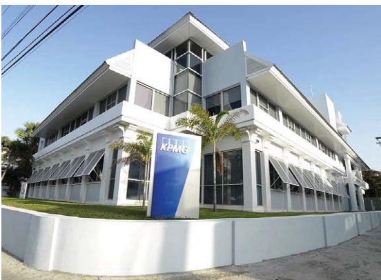
Hastings Office Centre 1 Hastings, Barbados
