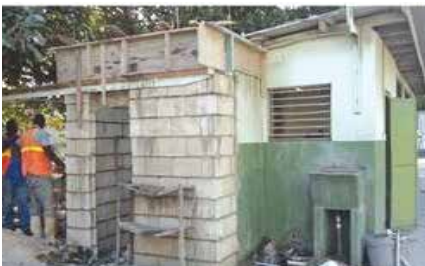
Truck Drivers' Washroom at CCCL, before and after
