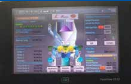
Raw Mill Control System
