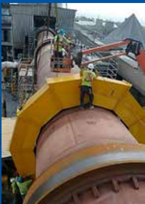
Kiln Shell Replacement
