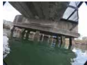
T&T (L-R): Traffic Management, Kiln 3 Shell Replacement, Jetty Pier Upgrade
