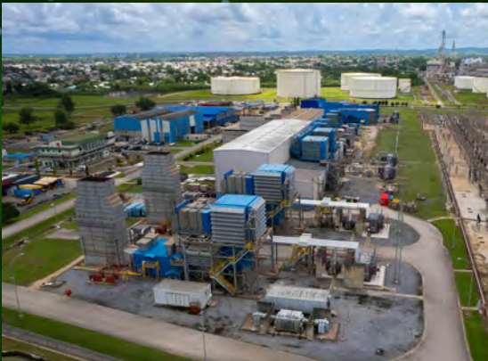
PowerGen's Pt. Lisas Power Station
