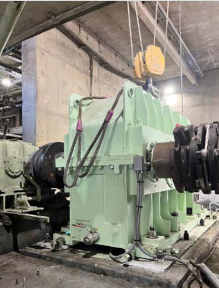
Cement Mill 3 main drive gear box installation
