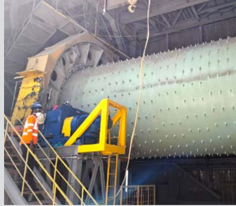
Cement Mill Repairs - Shell Change
