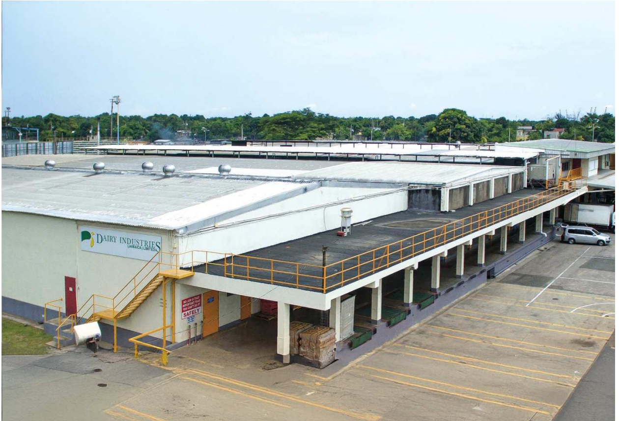
The Dairy Industries (Jamaica) Limited (DIJL) manufacturing facility, located in Kingston, Jamaica.
