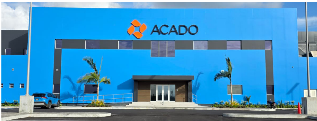
Acado Guyana's new warehousing and logistics hub
