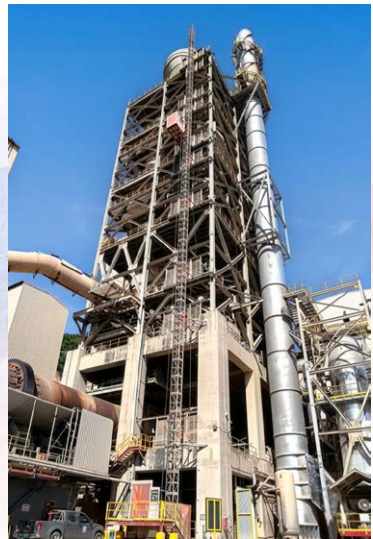
Jamaica - Kiln 5 Stack Replacement
