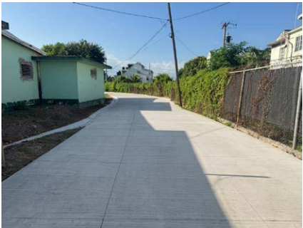
Calabar High School Road and Drainage Improvement project (Jamaica)
