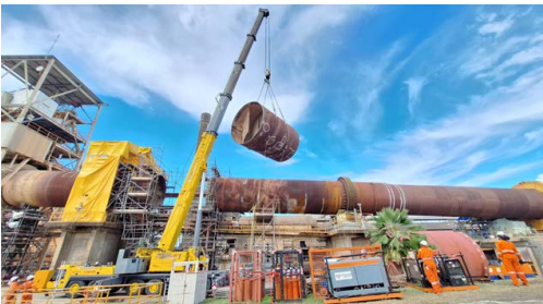
Kiln 3 Shell Replacement - Trinidad Cement Operations
